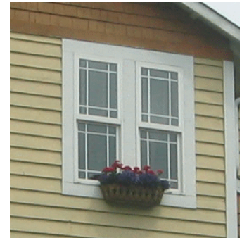
Window with trim OK
