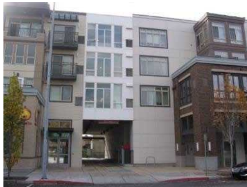
Example of a drive-through within a structure
