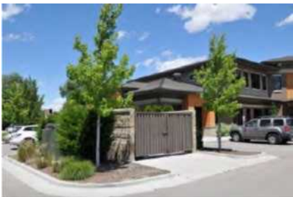
Well-designed service enclosure example.
