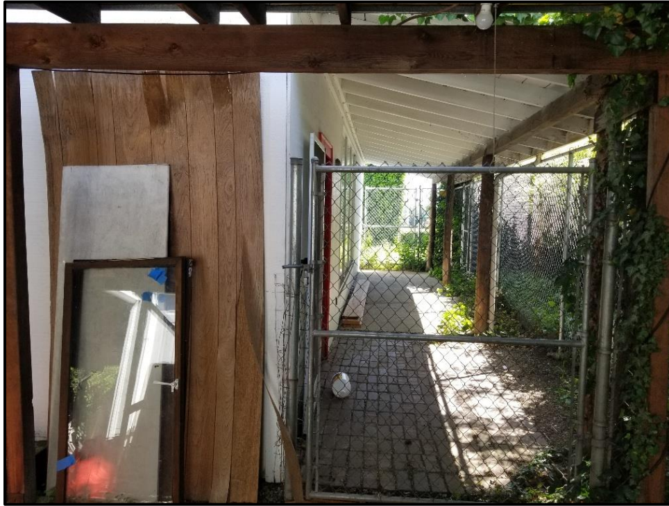
15. Interior view of the eastern boundary.
