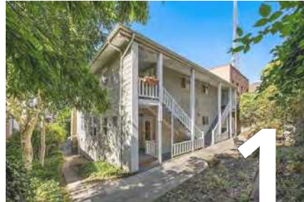
Cherry Court Condominiums Seattle, WA
