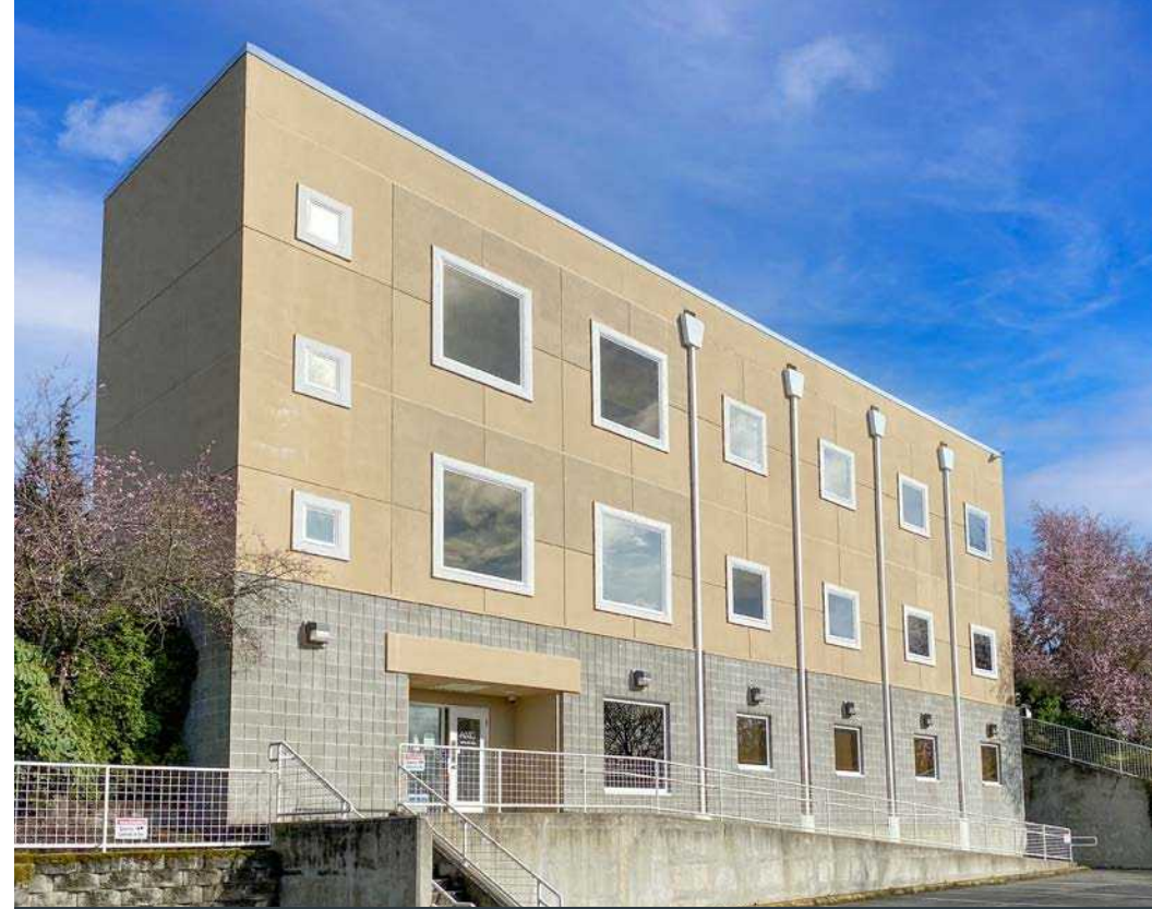
LOWER LEVEL ENTRANCE
