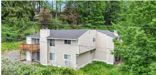
10th STREET APARTMNETS
