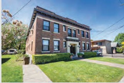
Riverside Apartments 1003 N 1st St, Renton, WA 98057
