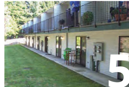
Lighthouse Townhomes 23524 100th Ave SE, Kent, WA 98031
