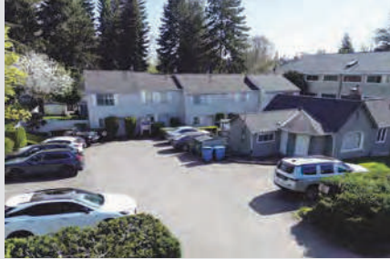
Shoreline Townhomes 1527-1529 NE 150th St
