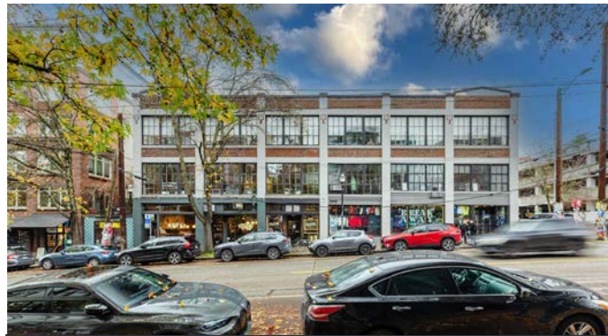
610 E PINE STREET MULTI-TENANT RETAIL & OFFICE
